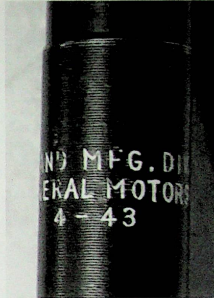
Above: Barrel marked Inland MFG. Division General Motors 4-43
